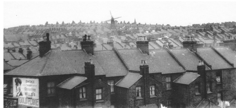
Terrace houses in the Delce area, built around the turn of the 20th century, showing the windmill at the top of Cossack Street.
