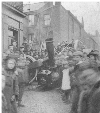
Accident to a Corporation roller in Cossack Street; 28 March 1908.
